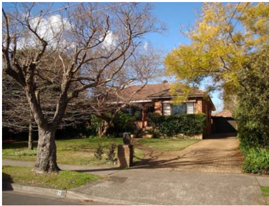
Image 6 34 Highlands Avenue, substantial Inter War house
